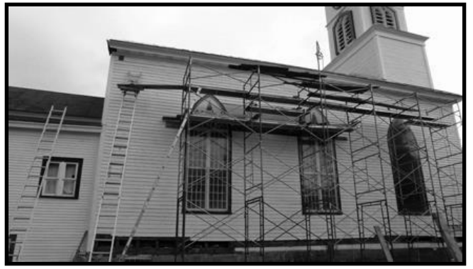
Closing up the top of the west wall.
