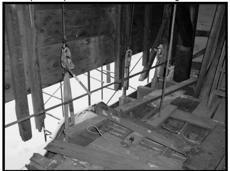
Girt removed. Rafters suspended by cables.
