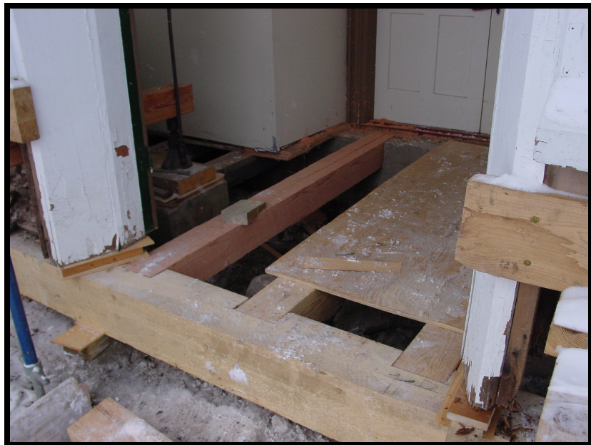
New 10 X 10 sill spans the entire width of the tower. New floor joists in the entryway.
