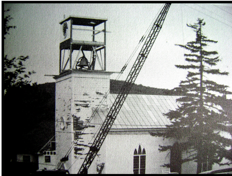
1985 reconstruction of top two sections of the tower. One clock face and the bell have been set in place. Also note new standing seam roof.
