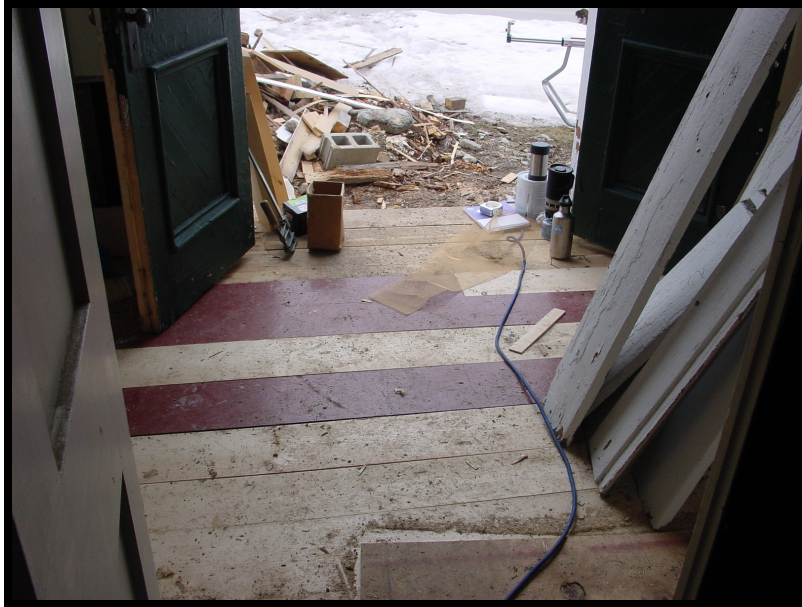
New floor. Red Boards are from original floor.
