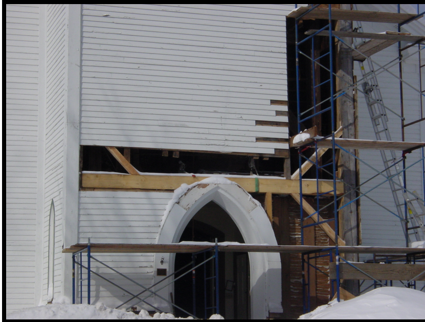
New plate with braces attached to new right front corner post. New vertical studs/post would be sistered to existing.
