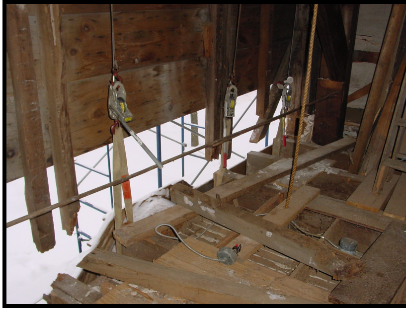
Void where the remains of the old plate/girt above the door were removed. Joists/rafters suspended by cables. Posts/studs and bracing held in place only by sheathing.
