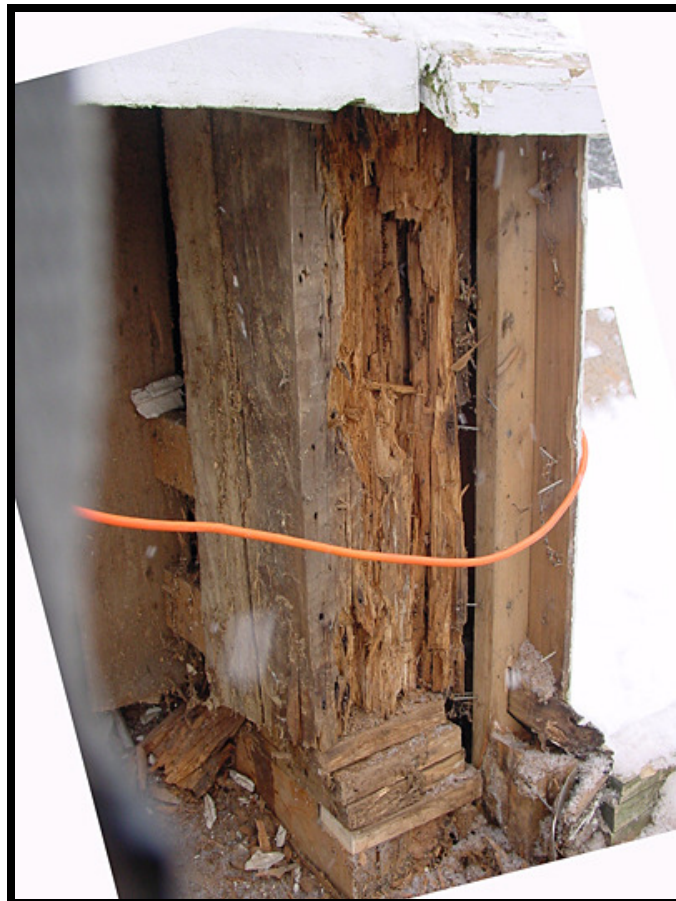
Extensive rot at bottom, of the front right post.
