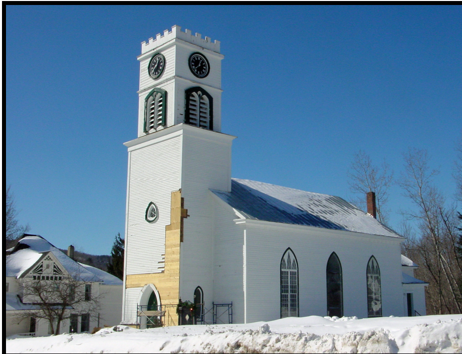
Late March 2011. New sheathing installed after urgent structural repairs (above) were completed. Additional joinery completed inside shortly thereafter.
