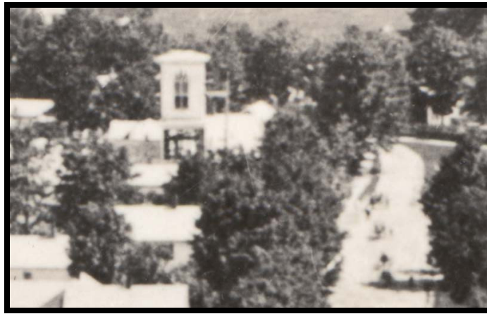
Union Church circa 1872. Tower being built, or retrofitted with clock and bell. Note the lancet window in the tower and the absence of the crenellation at the top.
