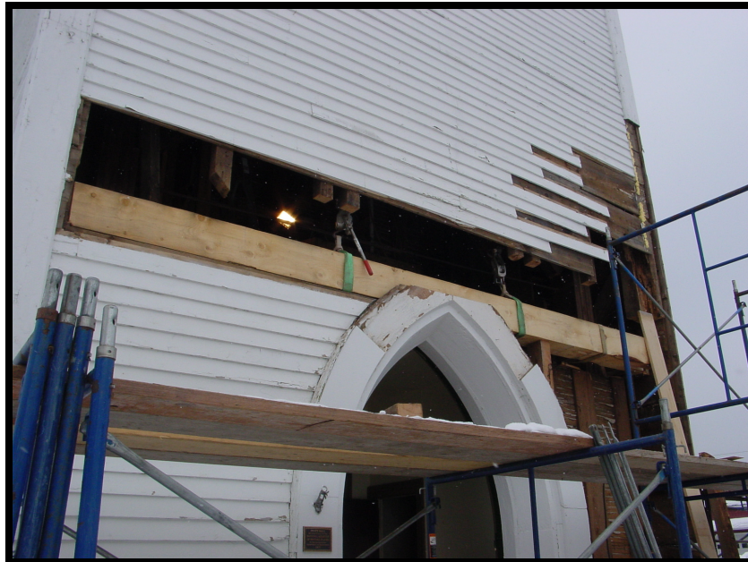
New plate hoisted in place.
