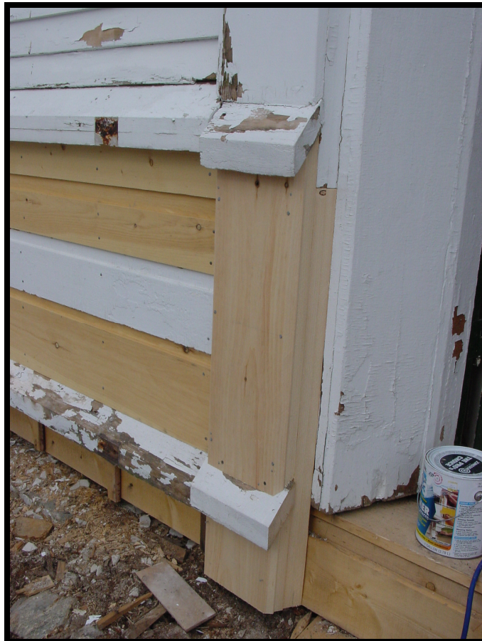
New siding and trim detail.
