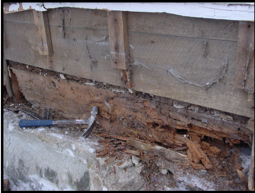
Exterior of front sill to the left of the door. Central portion of sill had disintegrated. Right portion of sill was identical to the above.
