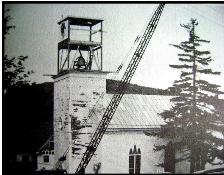
1985 reconstruction of the top two sections of the tower. One clock face and the bell have been set in place. Also note new standing seam roof.
