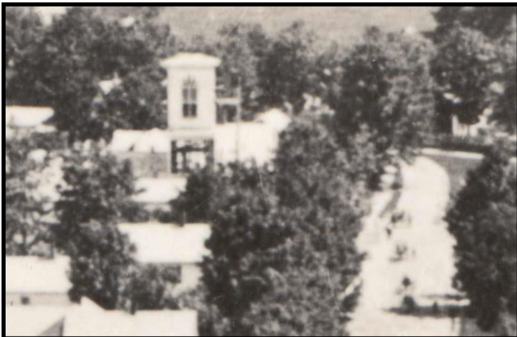
Union Church circa 1872. Tower being retrofitted with clock & bell. Note the lancet window and the absence of crenellation.
