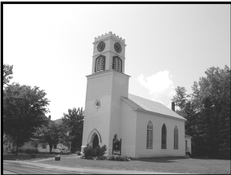
Structural Repairs Complete Pratt Hall June 2011
