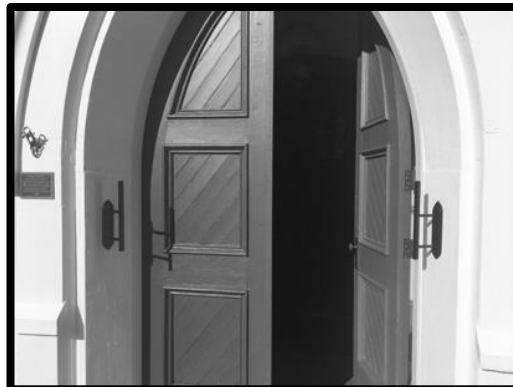
New Grab Bars Installed
