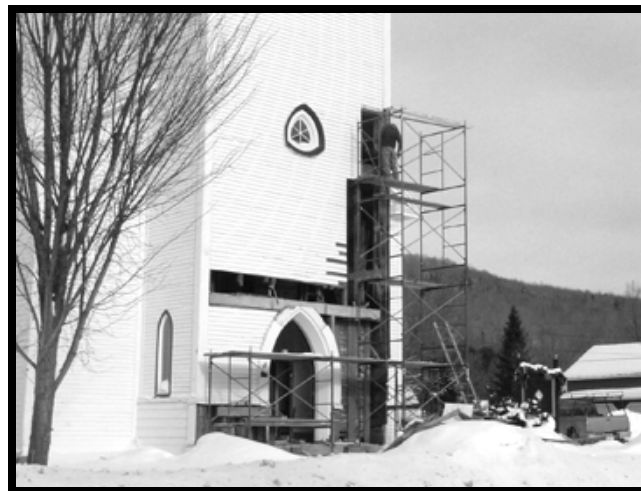
Restoration In Progress
